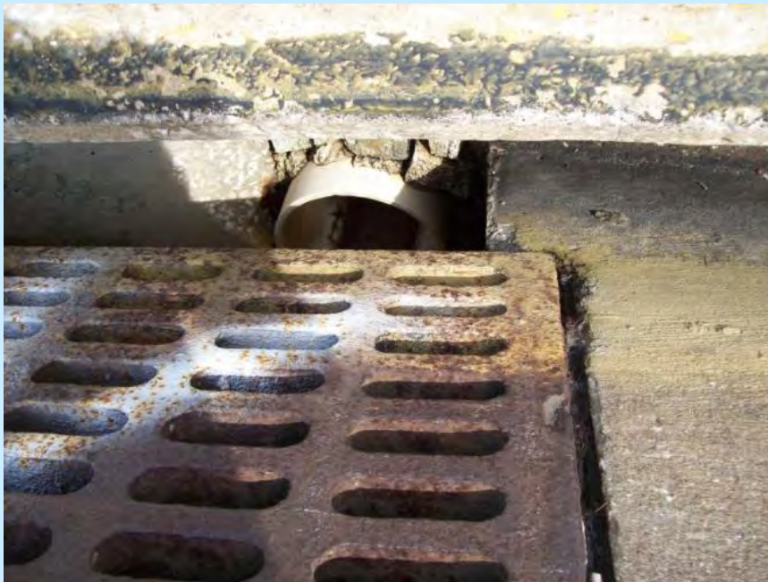
Unknown pipe into storm sewer inlet
